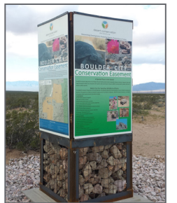
Gabion kiosk constructed along Route G in the BCCE.
