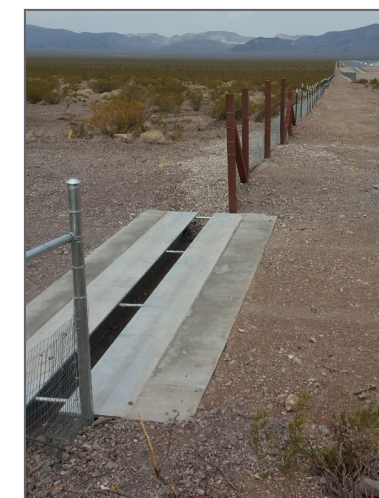
New desert tortoise guard constructed at an Energy Zone access point.
