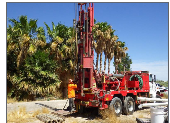
Equipment used to install piezometer groundwater monitoring wells.
